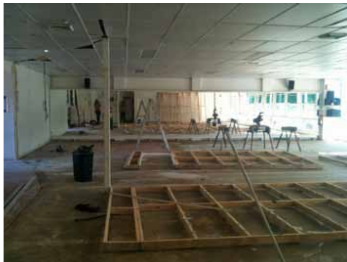
Image 1: Dance Central in Phillip January 2012 - a commercial studio stripped back to bare concrete floors before a sub-floor is installed for the dance surfaces. Photo Dance Central
